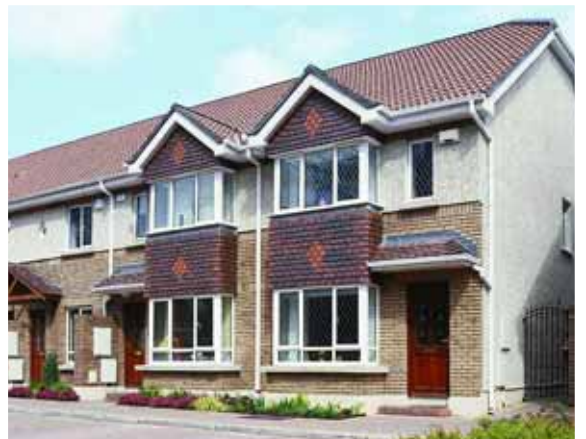
Ashtown Residential Development, Co. Dublin
